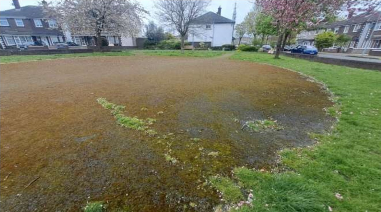
The amenity area in Beechpark Court - Coolock was powerwashed to remove the moss.
